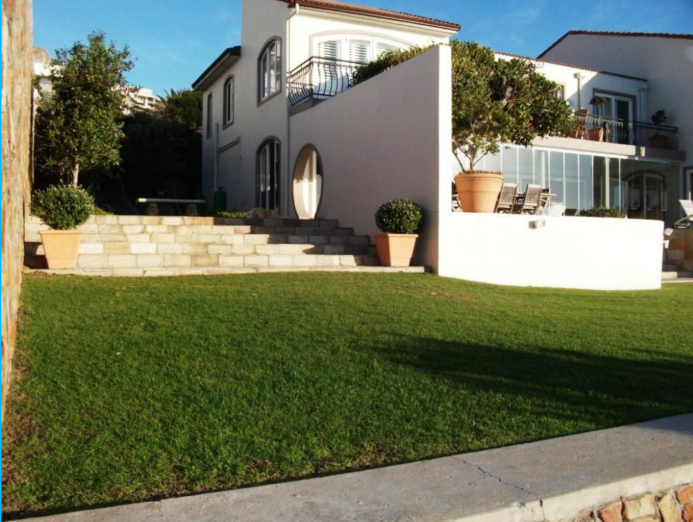
PLATE 1: THE EASTERN PORTION OF THE PROPERTY, VIEWED FROM THE SEAWARD/ NORTH-WEST BOUNDARY WALL, FACING SOUTH-EAST. THE PORTION OF GARDEN SEEN HERE WILL REMAIN UNAFFECTED BY THE WORKS AND WILL BE HOARDED OFF FROM THE CONSTRUCTION AREA.
